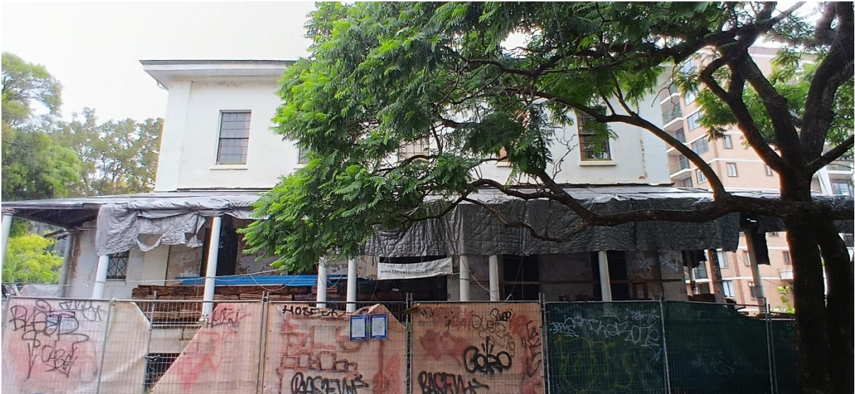
Figure 2: Front of Cleveland House viewed from Bedford Street facing south
